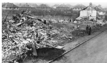
Bomb damage on Wickenden Road, Sevenoaks
